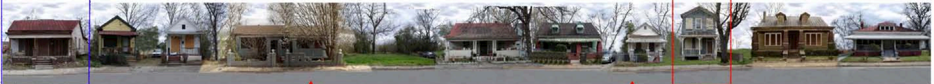
East Pine Street: Pre-construction
