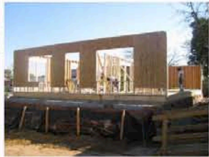
1218 Pine Street: Construction
